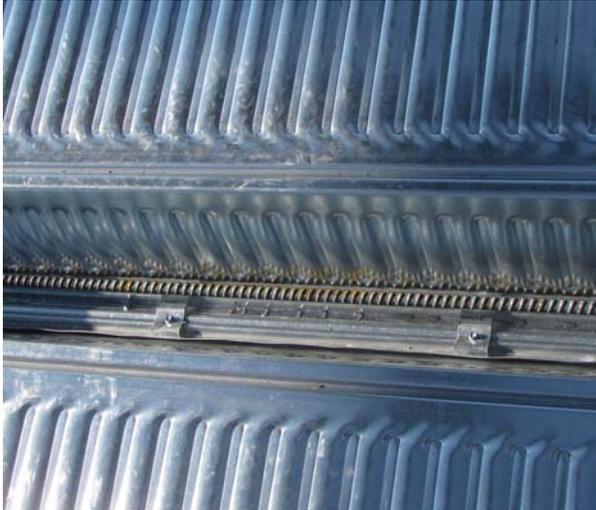
Figure 5 - Side lap washers visible under shifted rebar.
