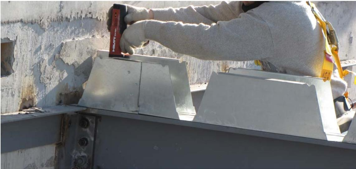
Figure 2 - Installation of end closures.
