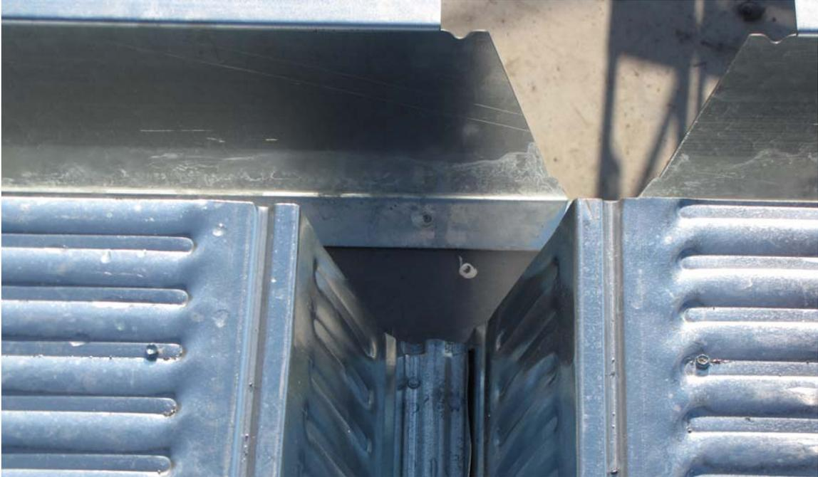
Figure 3 - Attach deck to support.
